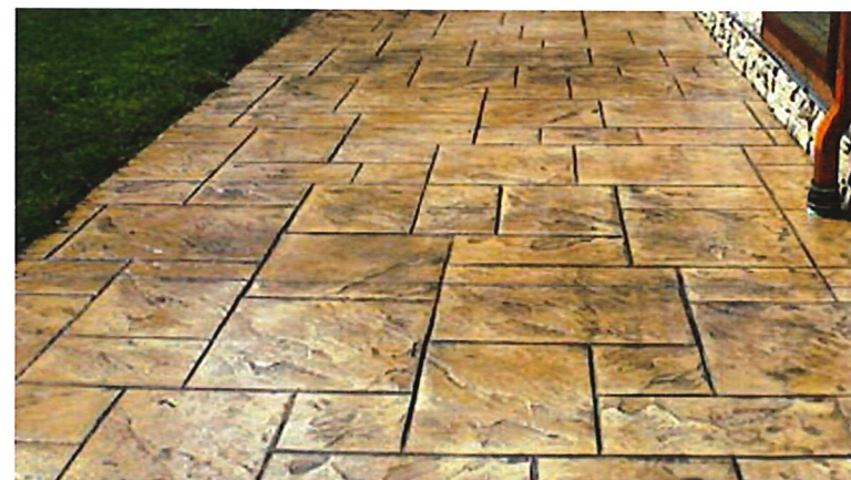
Stamped Colored Concrete Plaza Paving
