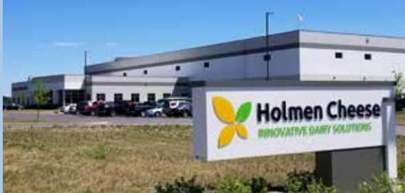
The above example provides a potentially acceptable use of concrete-panel using horizontal color bands and panel scoring to add architectural merit.
