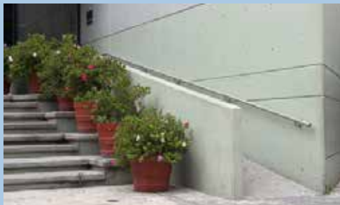
The ADA ramp is incorporated in the stair entrance, meeting the needs of all users.
