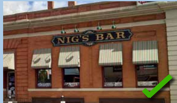
GOOD DESIGN. This sign is placed well within the existing architectural features (centered on the brick inlays and above the window/awnings, but below a cornice line).
