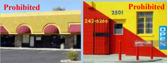
Examples of prohibited use of fluorescent / bright color as the primary facade color.
