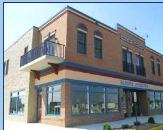
Example of a secondary facade continuing the design quality, material palette, and color palette of the primary facade. Note the change of material at an architectural element (protruding building plane).
