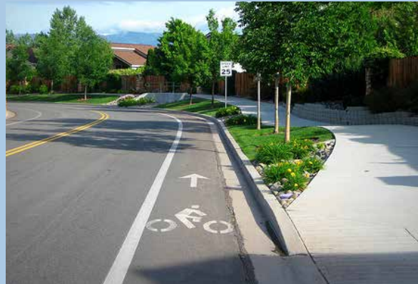
An example of road with a painted bike lane along with a landscaped sidewalk terrace.
