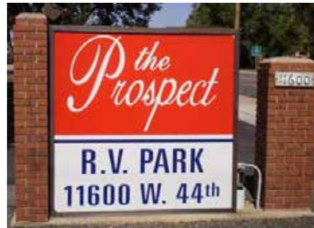
BAD DESIGN. Lack of overall composition between brick pillars, conduit visible, no base to the sign, no base landscaping, and excessive large text.
