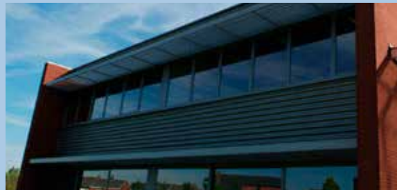
An example of a building using a high-quality decorative metal product as an accent material on a non-street facing facade.
