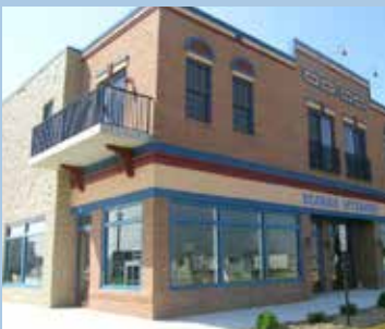
The example on the left shows the continuation of the front facade's design and materials to the side street, terminating at a change in the building plane.
