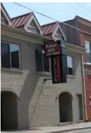
BAD DESIGN. The projecting sign is placed in front of a window while an alternative location is available. The mass of the sign is distracting to the overall building.
